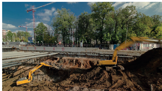
Figure 1 – Mechanized open-cut trenching – Bottom-Up Method
